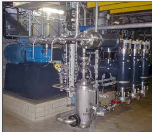
FELUWA MULTISAFE® double hose-diaphragm pump Example application: TG 130 – 3 DS 35 Triplex, single-acting pump: 5 to 20 m 3 /h at 35 bar and 30 °C Medium: 70 % hydrofluoric acid solution Media-contacting metal components lined with PTFE and hose-diaphragms made of PTFE
