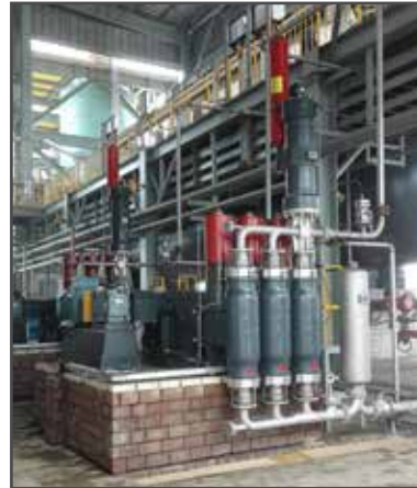
FELUWA MULTISAFE® double hose-diaphragm pump Example application: TG 135 – 3 DS 100 Triplex, single-acting pump: 24 to 47 m 3 /h at 70 bar and 100 °C Medium: aggressive and abrasive chemical catalyst Media-contacting components made of 1.4410 (Super Duplex) and hose-diaphragms of EPDM
